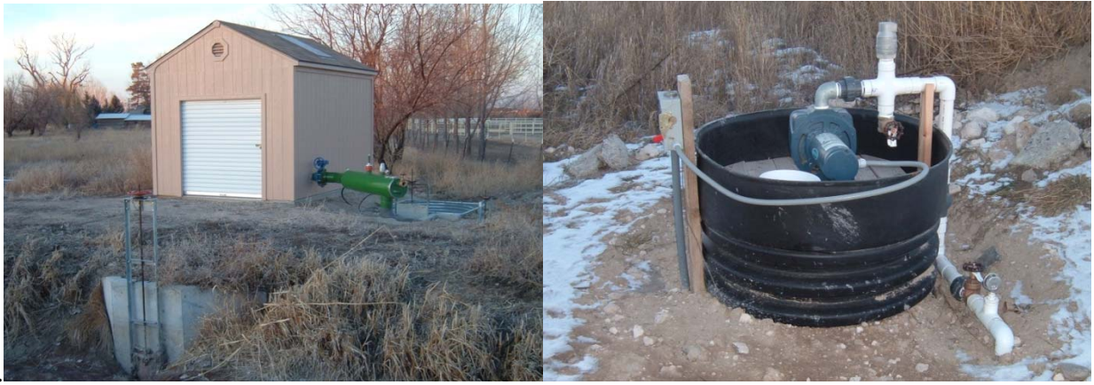
Figure 10. (left) Head gate, inlet screening and pump house for multiple-pump subdivision irrigation system. Capacity = 10 to 450 gpm; (right) pump sump and outlet for a two-user pumping system. Capacity = 20 to 40 gpm
