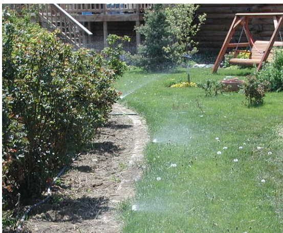
Figure 2. Pop-up half-circle spray heads. Head-to-head spacing is 10 feet.
