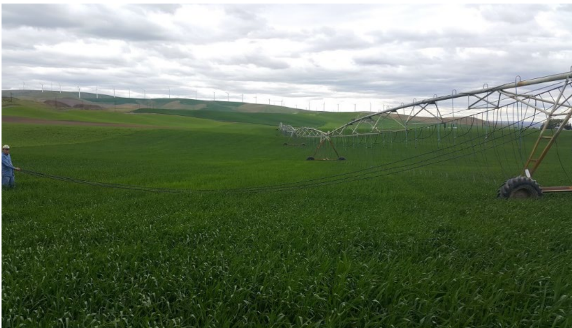
Figure 61. MDI installed on a center pivot while retaining the sprinklers for switching between MDI and MESA. The driplines on the outside spans of the pivot are longer since it covers a larger area in the field. Although the crop is wheat, the MDI system is set up for taller crops.
